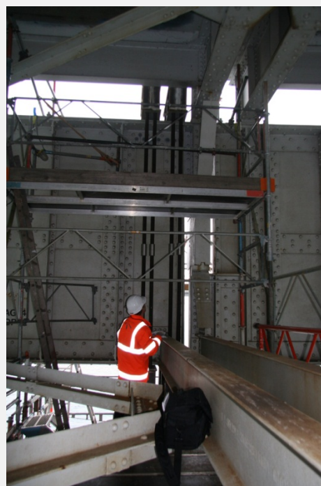
Inside the bridge during the repair
