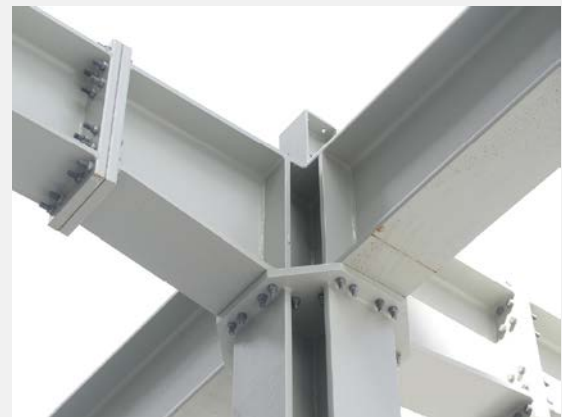
Fig. Bolted structural steel joints
