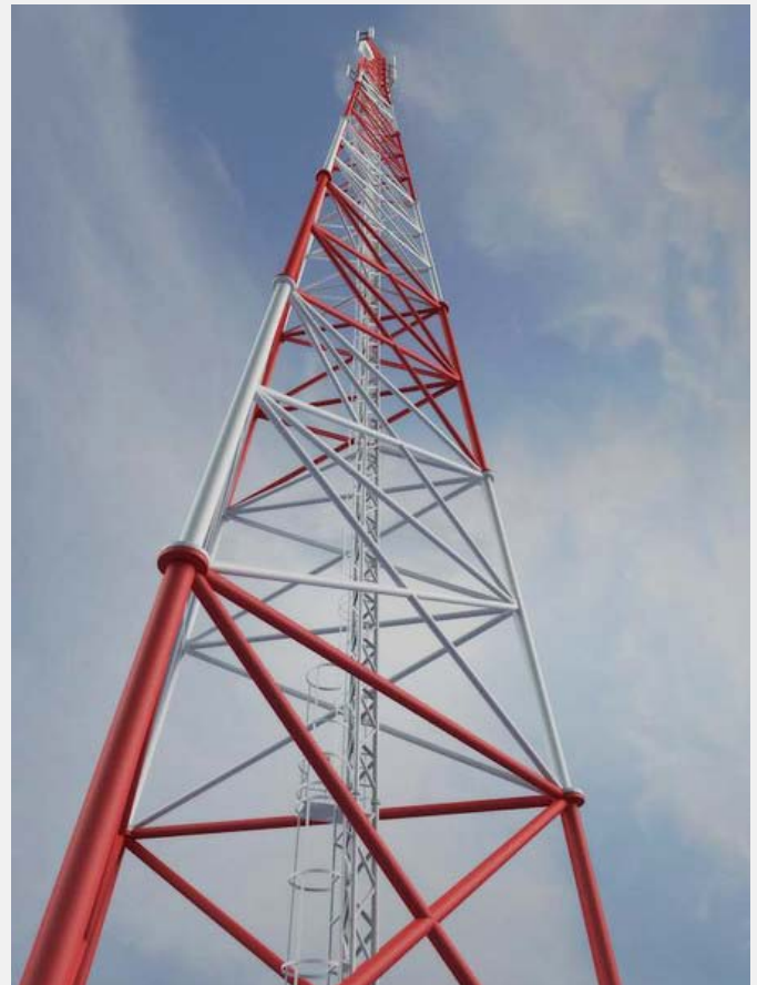
Example of the structure of a telecommunication tower. The wind loads on the tube-shaped elements are affected by scaling effects, which makes the design of suitable wind tunnel models challenging.
