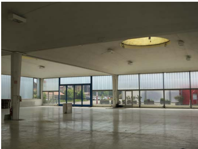
Factory building covered by rectangular shells. Designed and build by Heinz Isler 1954.
