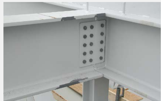
Fig. Bolted structural steel joints
