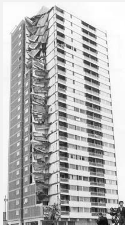
Progressive collapse due to insufficient robustness (Ronan Point)
